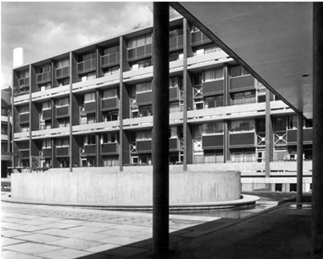
2/ Perimeter wall in 1962
